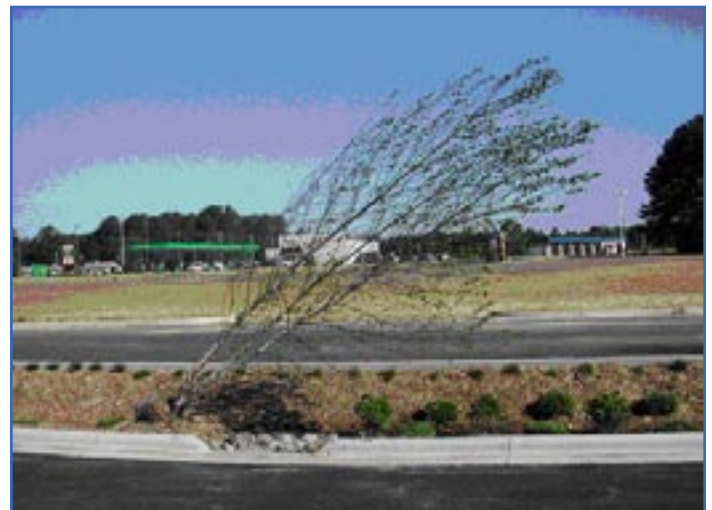
FIGURE 2. While River Birch ( Betula nigra ) typically grows well in bioretention cells, saplings need to be staked during the first year to keep them from being blown over in hurricane-prone North Carolina.
